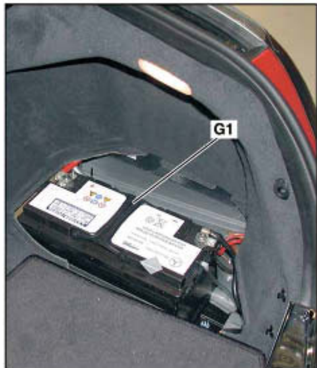
G1 Power supply battery on right side of trunk
